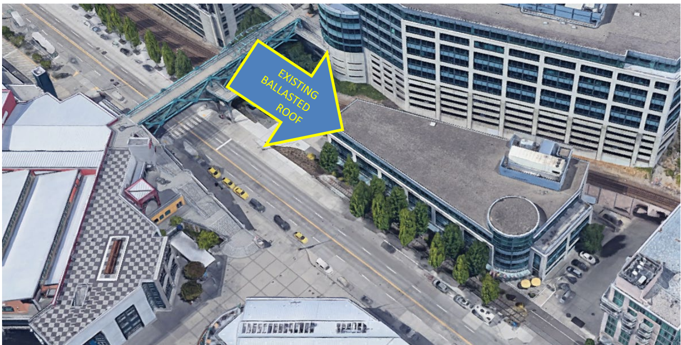
Figure 1. WTCW Roof Replacement Project
